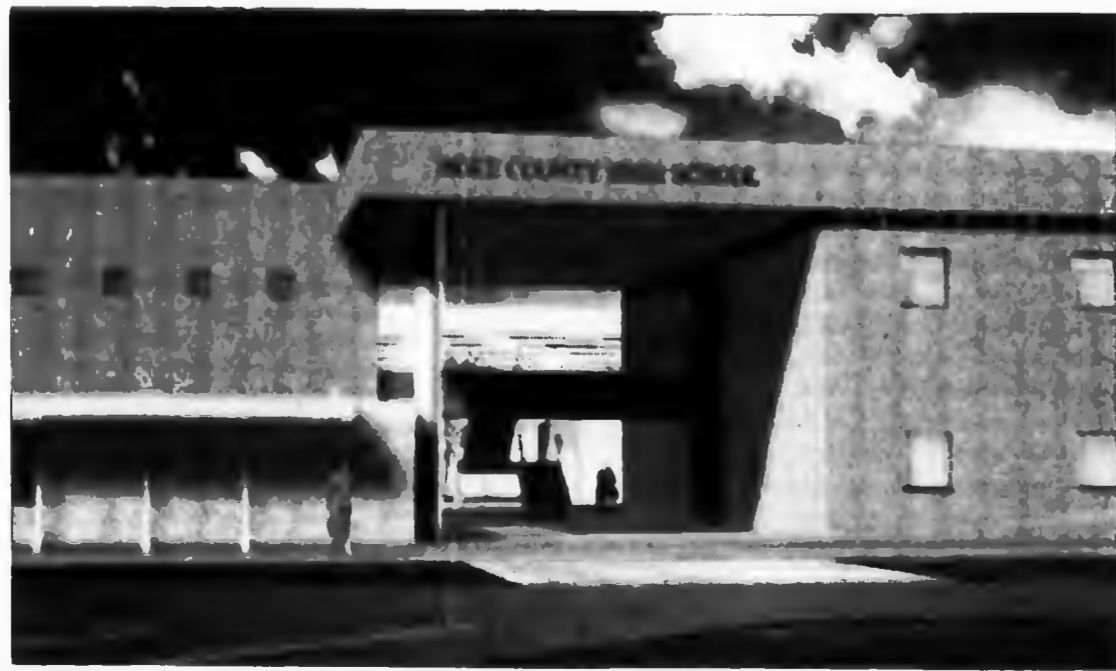
Architects' drawing of expansion under construction on the MacDonald side of Hoke High School.
