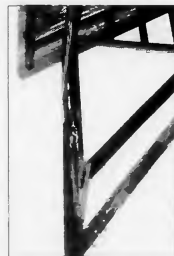
Workers were under this shelter when lightning struck. The bolt cracked an 8 X 8 timber (left) supporting the roof of the shelter in its upper left corner (right).
