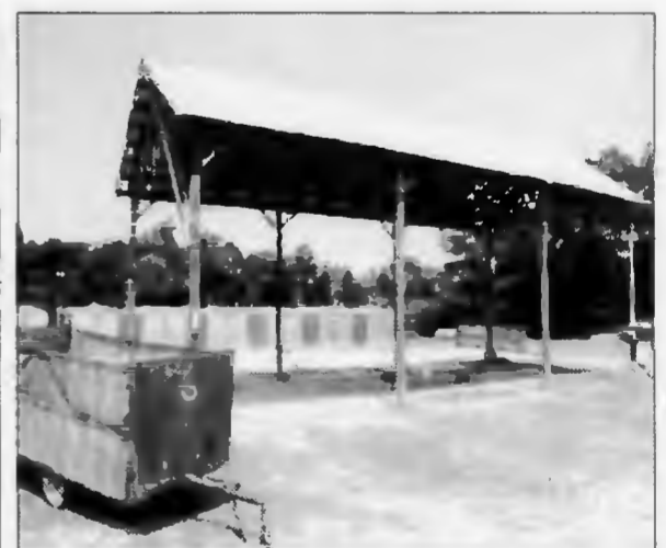
Workers were under this shelter when lightning struck. The bolt cracked an 8 X 8 timber (left) supporting the roof of the shelter in its upper left corner (right).
