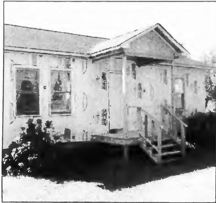
The Hoke home of Christine Henderson is undergoing rehab work.
