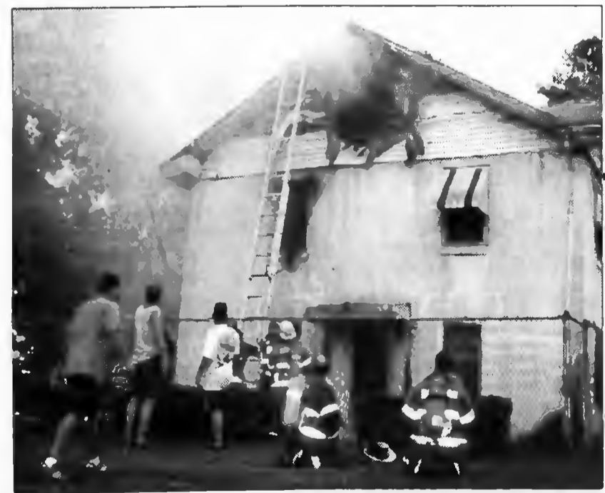
A storm on Saturday brought lightning and heavy damage to the home of Ivery and Ruth McNair.
