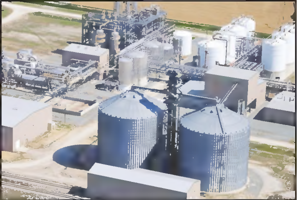
The Tyton Biofuels ethanol plant in Dundarrach.
