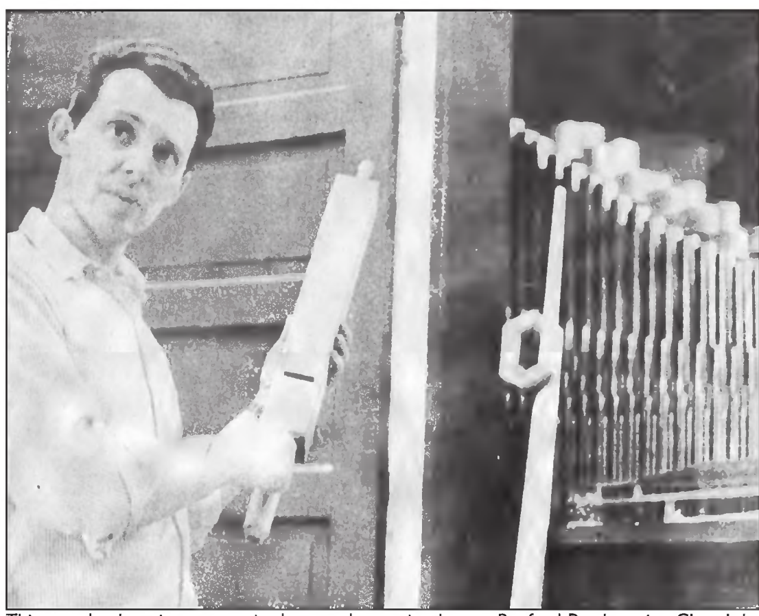
This wooden bass instrument is about to be put in place at Raeford Presbyterian Church by Roland Bonney, master of the art of installing a pipe organ. The nearly 2,000 pipes range from one and one-half inches in length to 16 feet. Installation is expected to be complete in a few days.
