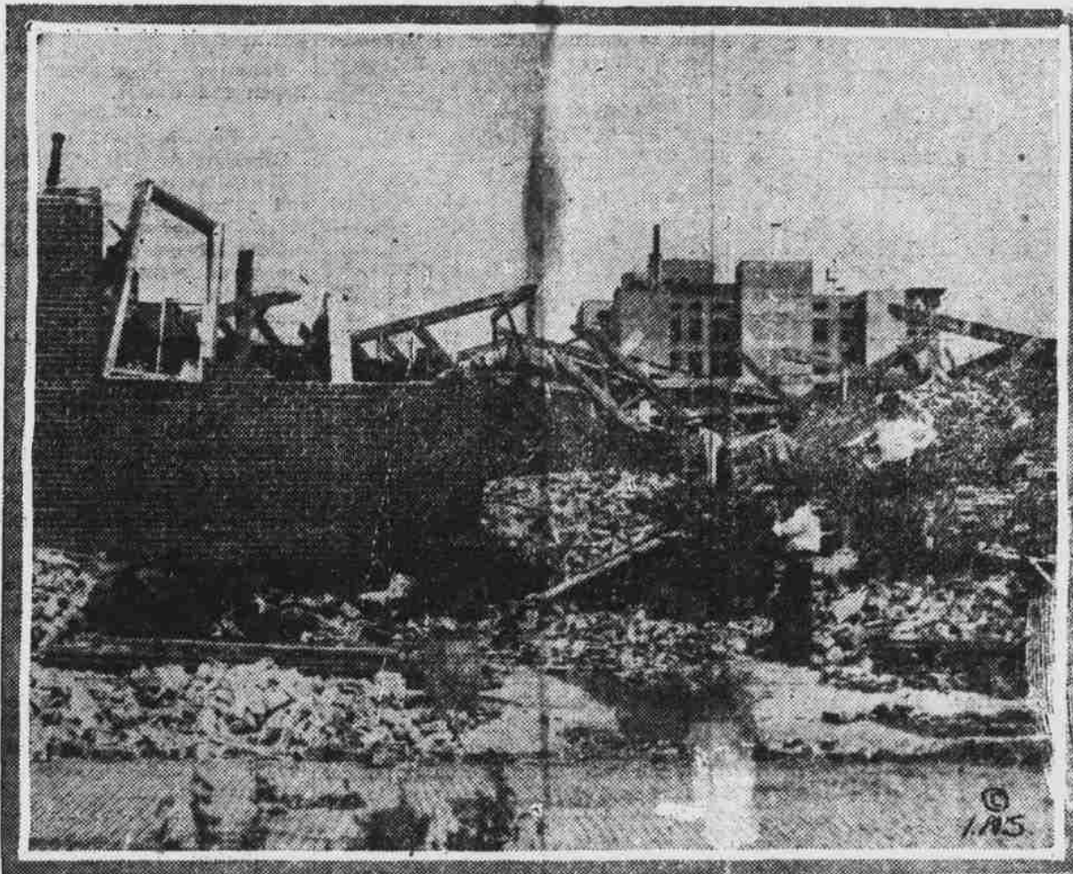
The West Indian hurricane that swept the Gulf coast on August 16, claimed a toll of more than two hundred lives and entailed a property damage that will run into tens of millions. Only the strength of the sea wall, which was erected for just such an emergency, and which stood fast in most places despite enormous pressure of wind and waves, stood between the city and such a catastrophe as visited it during 1900. With true American spirit the inhabitants are already busy rebuilding their damaged or destroyed homes.
