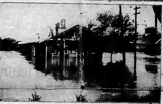
This picture shows the Southern Railway depot, entirely surrounded by water. The water, at its highest, stood about four feet above the platform of the depot. The contents of all cars standing on the siding, as well as all the freight stored in the depot, was greatly damaged. A force of men were put to work Monday after the flood, cleaning out the mud, which was nearly two feet deep.
