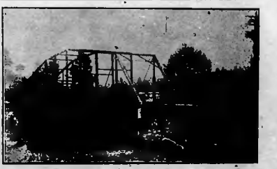
This big steel bridge, erected in 1913 by the sister counties of Surry and Yadkin, was swept away in the flood of July 15th. It landed only a few hundred feet below, but is tilted and warped so badly as to be of no value. The bridge was built at a cost of $4,500, and at the time of construction was considered safe. The destruction by water, compared with the previous high-water marks. The new steel bridge that is to replace the old one is 10 feet higher, and 510 feet in length, not including approaches, and will be equipped with a double drive way and a center walk way. The new bridge will cost about $20,000.
