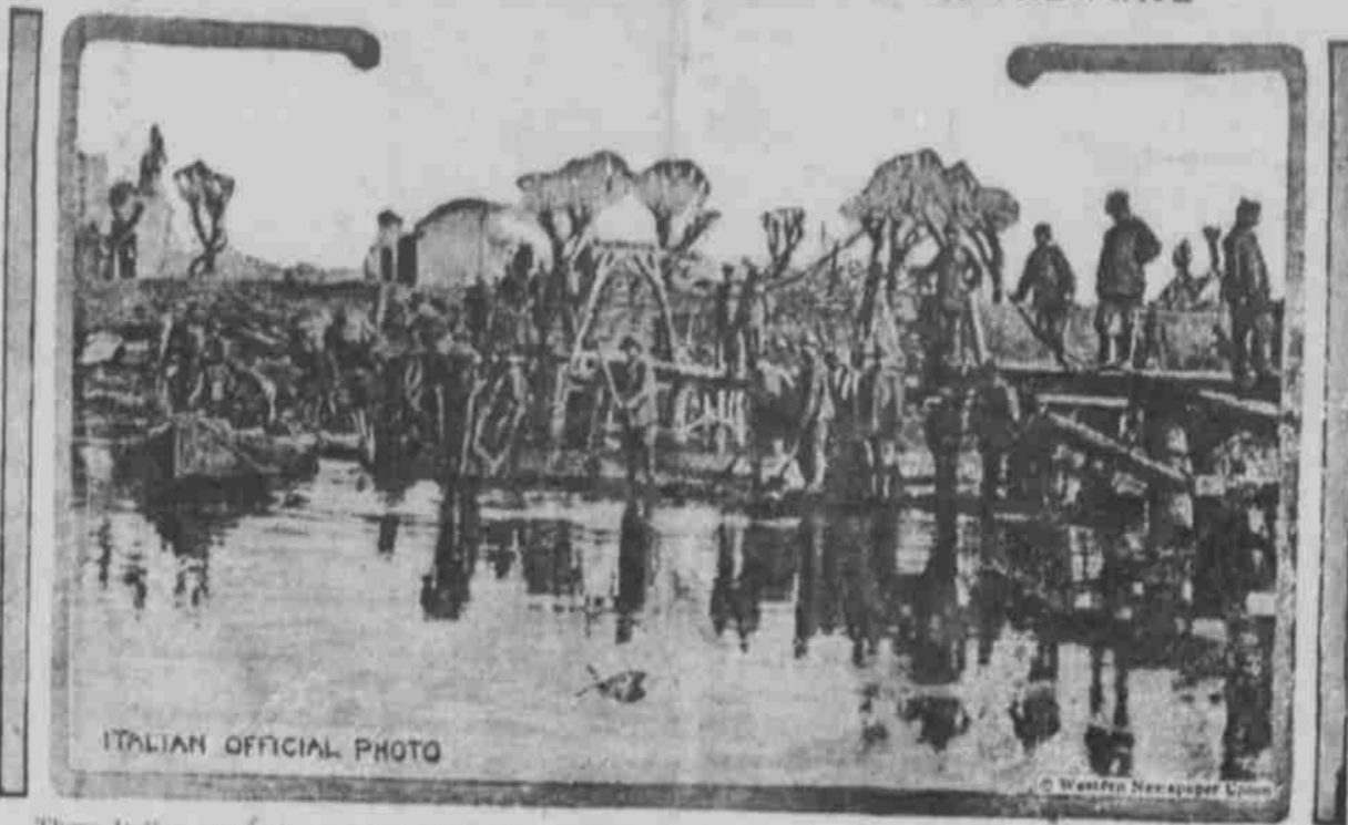
These Italian troops have driven back the Austrians on the Piave and are busy constructing a pontoon bridge to cross that river. The fighting on that front has been intense.
