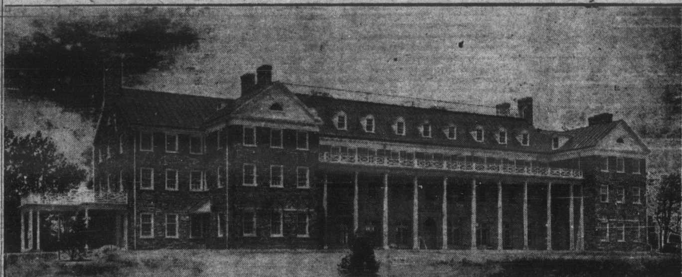
GRAYSTONE INN, MAGNIFICENT HOTEL LURED BY THE PIRE BREEZES ATOP THE BLUE RIDGE AT 3700 FEET ELEVATION WHICH IS THE SUMMER WHITE HOUSE OF NORTH CAROLINA WHERE GOVERNOR O. MAX GARDNER WILL SPEND THE SUMMER SEASON AT HIS OFFICIAL WORK FAR FROM THE HEAT OF THE LOWLAND CITIES.
