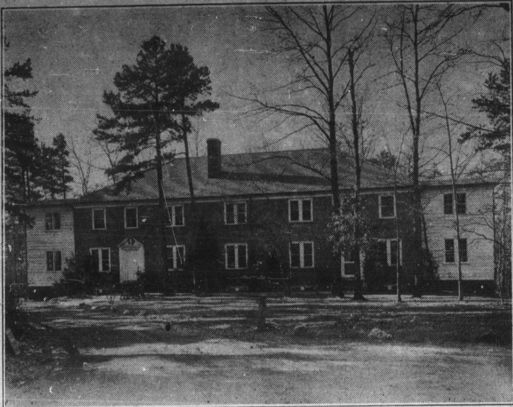
Above is a photograph of the Nurses' Home at Hugh Chatham Memorial Hospital showing the new extensions on the east and west sides which provide additional bedrooms, needed to take care of the increased staff of nurses required by the new hospital addition. This building is also the home of Dr. C. L. Haywood, Jr., hospital surgeon.
