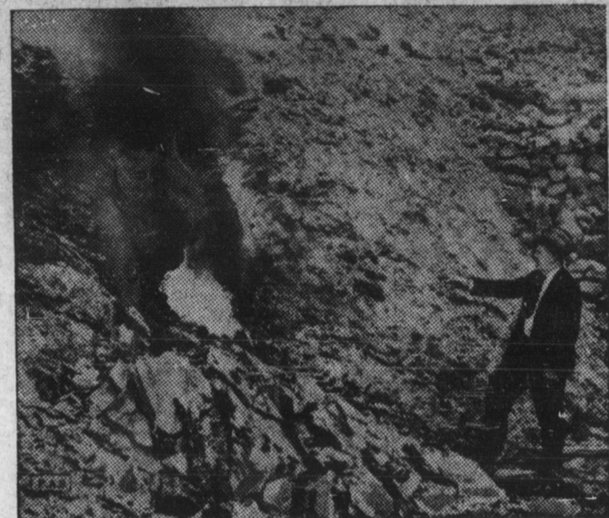
New Lexington, Ohio . . . The federal authorities' theory that the 54-year-old mine fire which has been raging with the force of a score of blast furnaces could be stopped by fighting it with wide tunnels of mud, has met its first test and proved successful.
