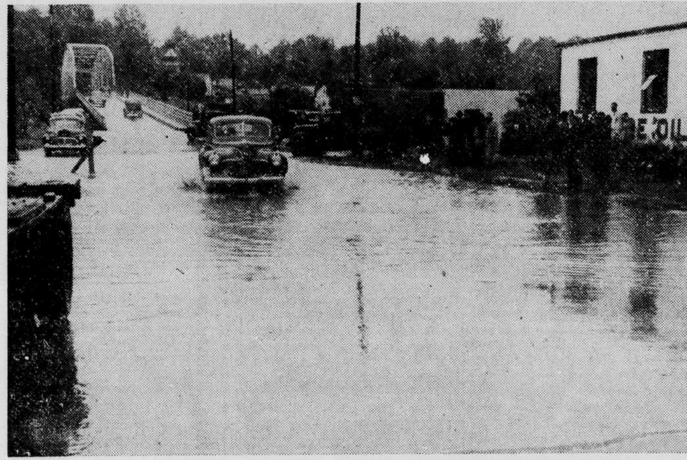
FLOODWATERS THREATEN ELKIN —The photos above were taken Saturday as the floodwaters of the Yadkin threatened to inundate the town. Top photo was taken from the old Elkin-Jonesville bridge and shows the Elkin Livestock Market flooded to a depth of several feet. Bottom photo shows an automobile plowing through the foot-deep stream flowing across the approach to the old bridge. The river reached a depth of almost 20 feet and destroyed hundreds of acres of crops along the valley. (Another flood picture on page 8, first section).
