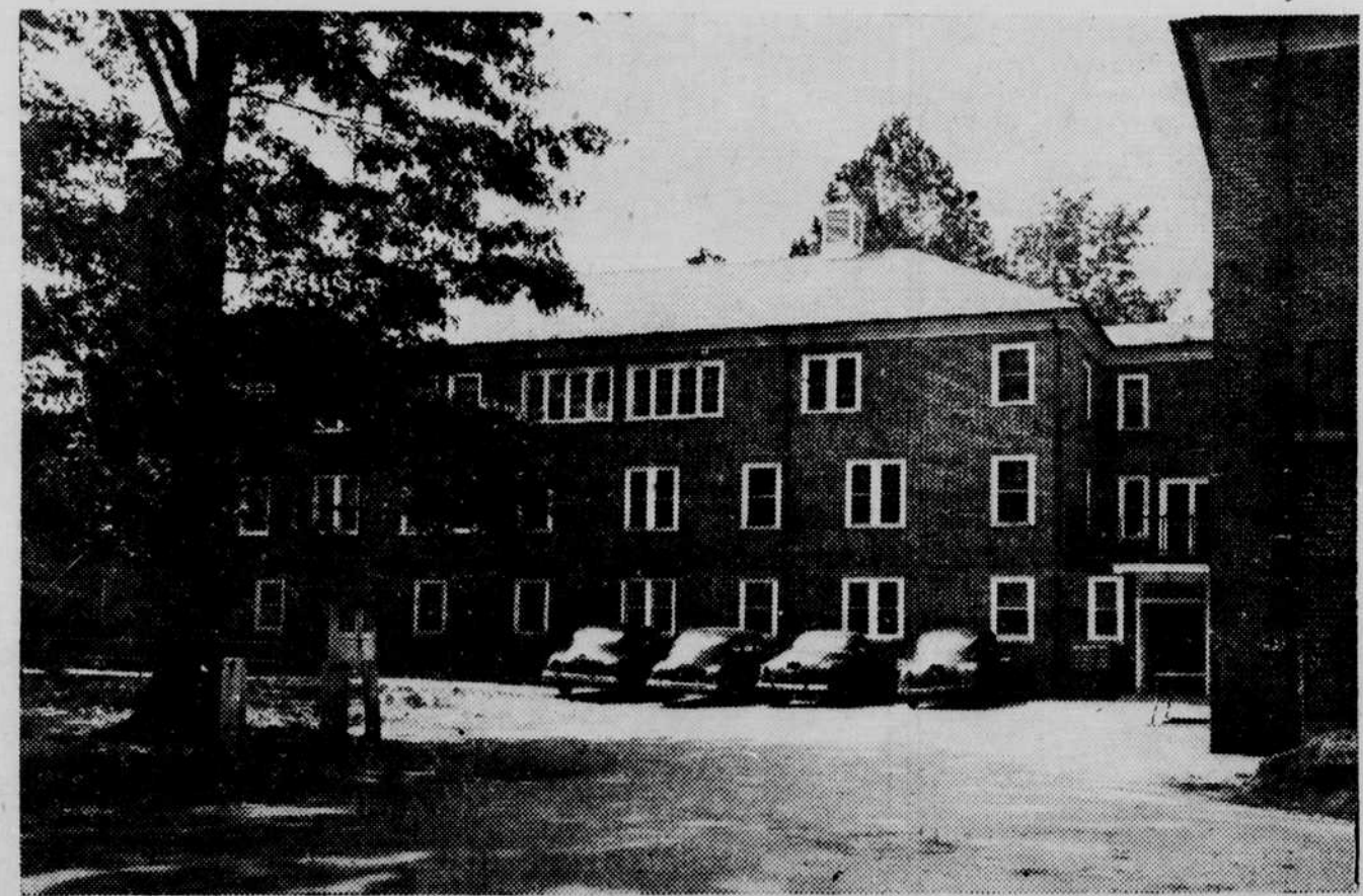
TO DEDICATE NEW ANNEX — Pictured above is the new addition to Hugh Chatham Memorial Hos- pital, which will be dedicated on May 27. The new addition will provide room for 16 additional beds as well as office and treatment rooms, and a new central heating plant which will serve the entire hos- pital. (PHOTO BY REDMON)
