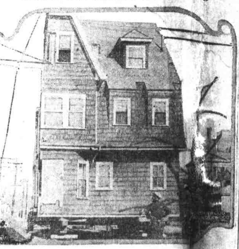
This half of a three-story house was photographed while being moved along Greenwood avenue, Newton, Mass. The section, weighing approximately 30 tons, was being moved from the residential section of Newton to a site one-quarter of a mile from its original spot.
