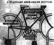
Note the enormous increase in the strain smaller sprockets and a 9-inch lower gear,
