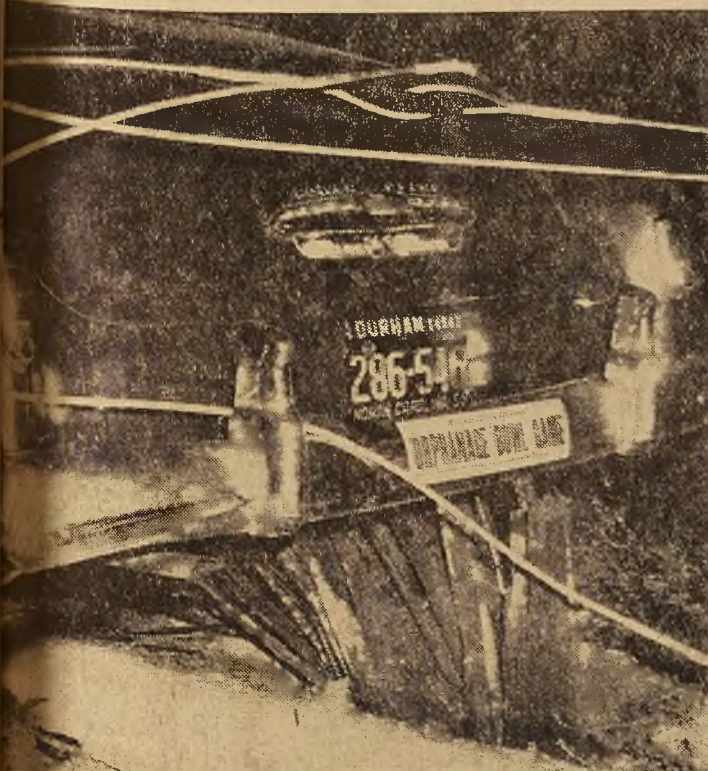
SHED OFF —The rear bumper of the Claiborne Hunsuckle auto rests on the stump of the 7,500-volt power line pole on Durham Road, which it sheared off at 6:50 p. m. last evening, plunging the town into darkness.
