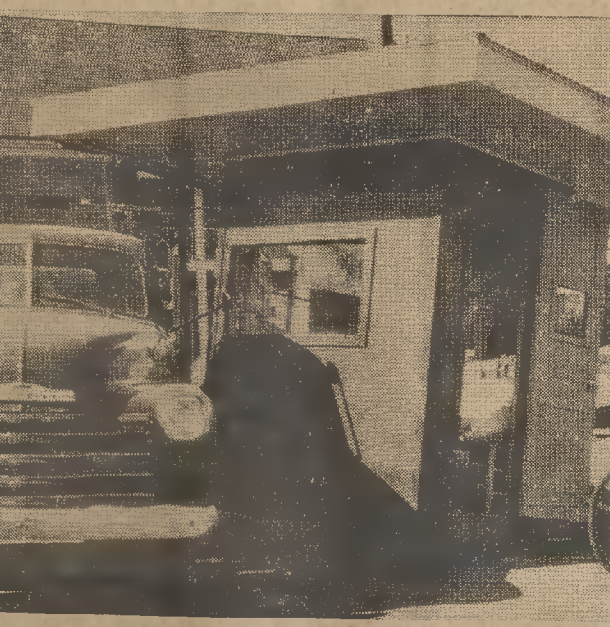
BUMP FOR A BOOTH —Davie Currie, attendant for the Chapel Hill Parking Association's downtown parking lot, got quite a jolt Wednesday morning as a truck bumped the roof overhang of his booth, jolting the building off its foundations. Damage was negligible. The driver L. W. Vick of Carrboro, reportedly misjudged a turn as he entered the parking lot.
