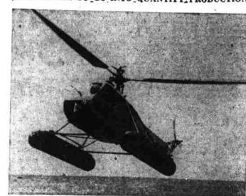
This Sikorsky type of helicopter, which will be built in quantity for the Army Air Forces by Nash-Kelvinator Corporation, peacetime manufacturer of automobiles and refrigerators, can alight on land, water, snow, thin ice, a rooftop or a parking lot. The craft can hover motionless in mid-air; descend and ascend vertically without forward motion and fly backward, sideways or forward with equal facility.
