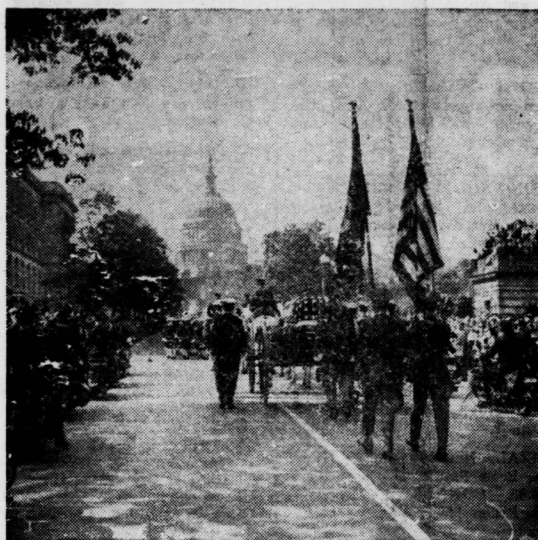
With the Capitol dome an imposing backdrop, the military procession, headed by the caisson bearing Franklin D. Roosevelt's body, winds its way down Delaware avenue toward the White House. The sad journey from Union station was viewed by millions. The presidential and U. S. flags bring up the rear.
