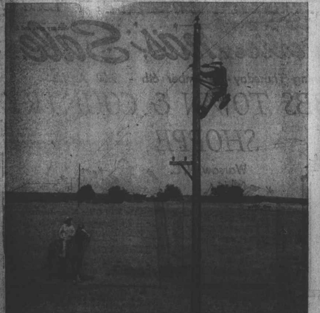
John McGuffin finally gets electricity in 1962, thanks to rural electrification
