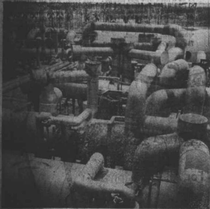
MAZE OF PIPES—A maze of pipes dwarfs Alex Cooke at CP&L's L. V. Sutton plant at Wilmington. Workmen flush these pipes with hydrochloric acid to clean them.
