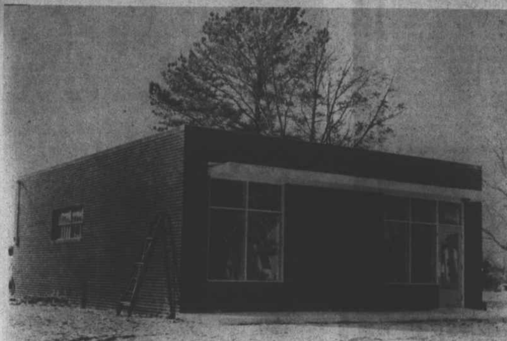
New $11,000 post office ready for occupancy at Teachey. Constructed by Ray McMillan and leased to the government.
