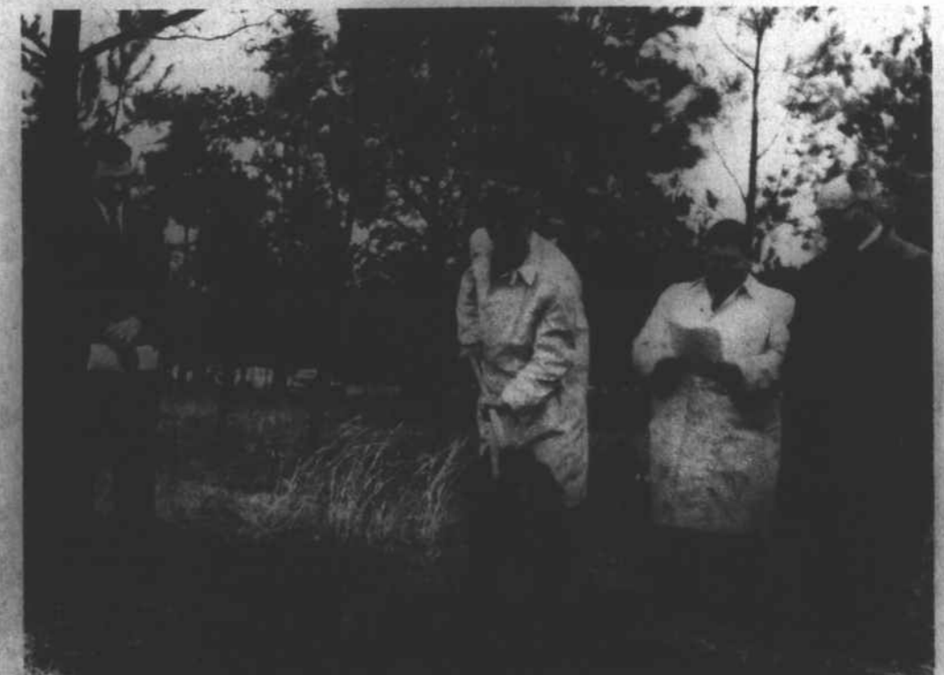
GROUND-BREAKING EXERCISES. Construction will begin shortly on a new Methodist Church in Beulaville on Hwy. 111 just inside the city limits. The new church was organized in 1958. Mayor Herman Gore (left) looks on as William B. Cutler, chairman of the building committee, breaks the ground. Rev. Foster Reynolds, pastor of the church, and Dr. R. Grady Dawson, district superintendent of the New Bern District follow the program. (Staff photo by James Campbell).
