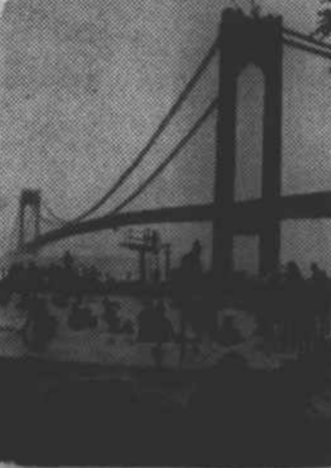
WORLD'S LONGEST BRIDGE . . . of a suspension type is almost completed. It is the Verrazano Bridge, which will connect Brooklyn and Staten Island with a main span of 4,260 feet. Prompt treatment of "strep" infections in the throat usually can prevent rheumatic fever and the heart damage it sometimes causes, says the North Carolina Heart Association.
