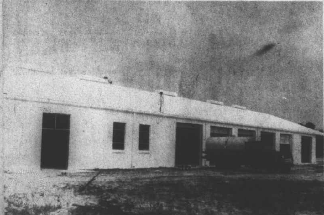
Duplin County's Garage is rapidly nearing completion, and plans are being made to occupy the new structure in the near future. The new building contains adequate and modern working space for repair purposes, a stock room, and two offices. Franklin Quinn, Cost Clerk, assisted by Jane Fields, will occupy one office, and the other will be used by Willard Brinson. Mr. Brinson is supervisor in charge
