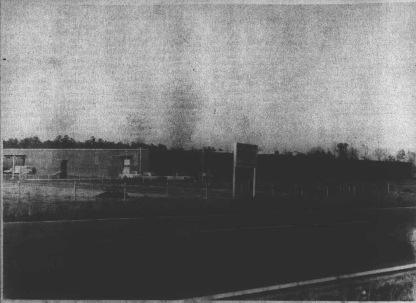
Reeves Brothers, manufacturers of Comfy Home products, is the newest industry to come to Duplin County. With 100,000 square feet of floor space in the plant, and more than two hundred employees, Reeves Brothers is a welcome addition to the county and to its economy. Reeves Brothers invites you to Open House Saturday, April 15.
