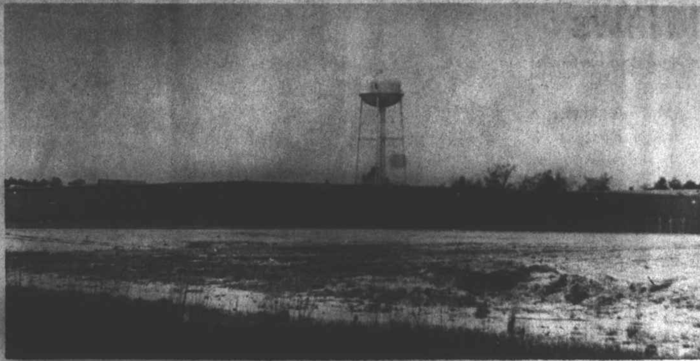
REEVES BROTHERS of Kenansville showing the 50,000 foot addition on back to the 100,000 feet already there. Reeves Brothers opened March 14, 1966 in the C. E. Quinn Store in Kenansville and moved into their new plant on June 28, 1966. They started with 45 employees and now have approximately 300 employees. Plant manager is Charles Ledbetter and Ralph Cottle is Personnel Manager. They both express appreciation
