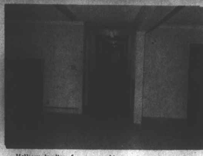
Hallway leading from assembly to classroom in educa- tional building.
