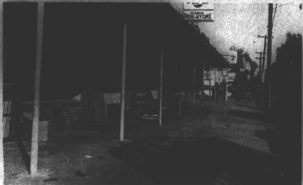
Fire swept this shopping center in Warsaw Sunday afternoon and left only the walls of Western Auto and Clarks Drug. A plate of plastic flaps in the Farmers Hardware and Merchandise window, which received only minor damage.
