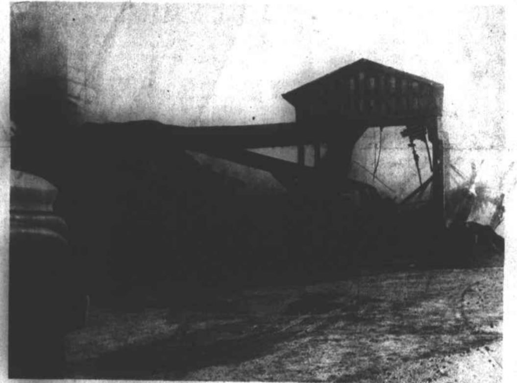
Fire destroyed the original section of Aycock Milling Co. in Wallace. An estimated damage of $75,000 was done to the southern section of the plant.
