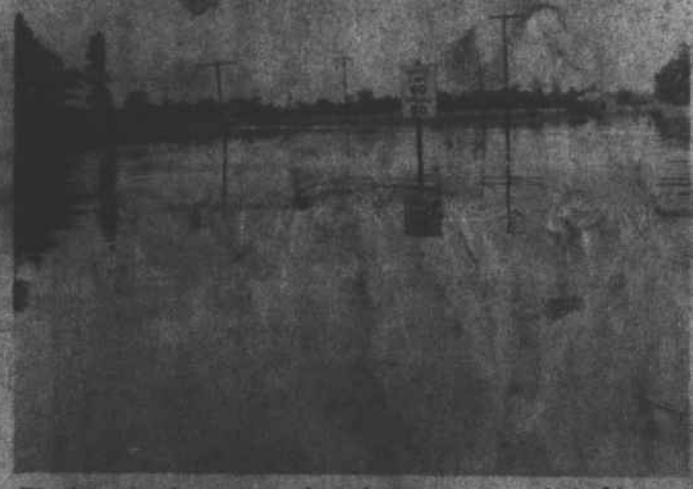
Flood water damages roads and cause a great deal of inconvenience.
