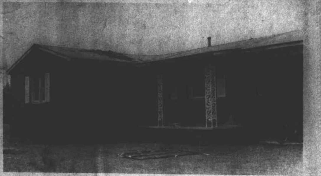
Rose Hill Fire Department extinguished a fire in this house early Sunday morning. Flammable materials were later found camouflaged in a bedroom closet.
