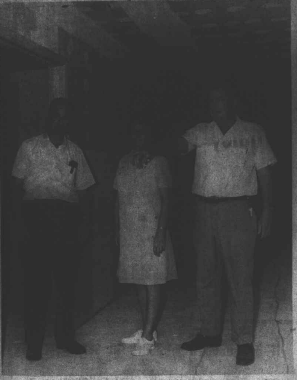
D. J. Fussell left with Carolyn and John Hall examine work on the latest addition to Whaley Rest Home in Kenansville, which is expected to be ready for occupancy early in October. Photo by Ruth Wells
