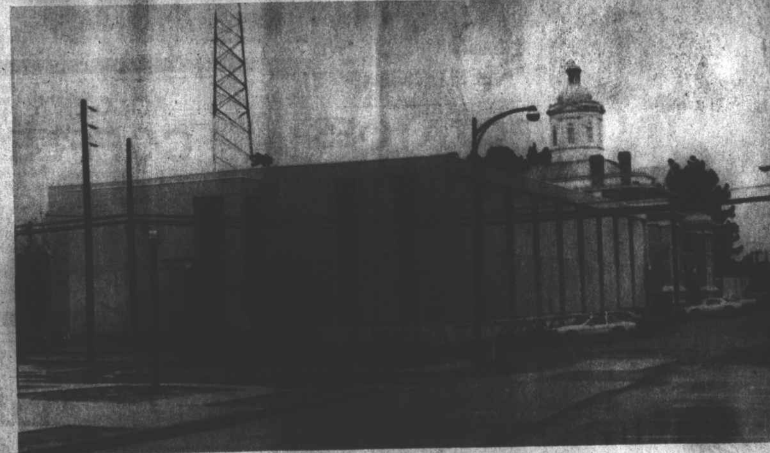
Duplin Jail And Courthouse Nearing Completion
