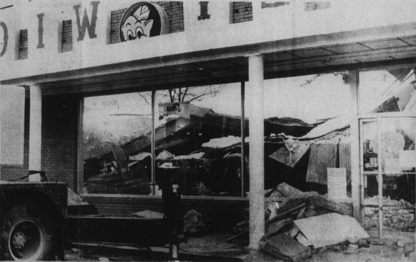
FAISON PIGGLY WIGGLY ROOF COLLAPSES - Late in the shopping day Tuesday, March 4, the snow-covered roof of the Faison Piggly Wiggly collapsed injuring four persons. Three store employees and a customer were rescued from the front of the building in the check-out area where the roof fell without warning. All except the customer, who was
