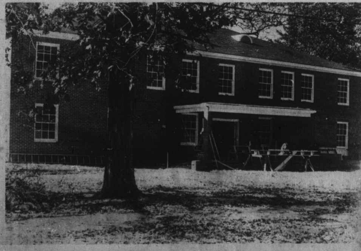
Renovations being completed at the Warsaw Medical Center.
