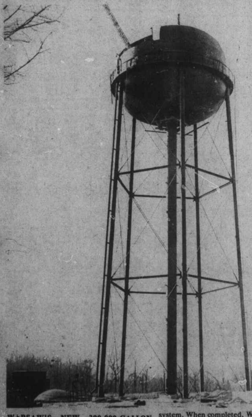
WARSAW'S NEW 300,000-GALLON WATER STORAGE TANK TAKING SHAPE
