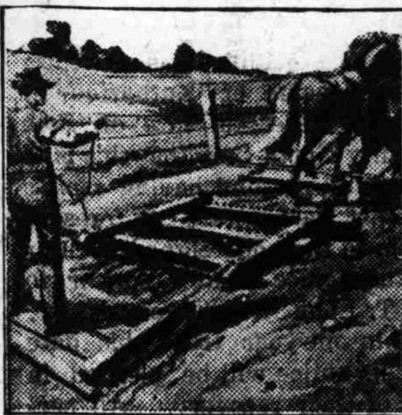
The Spiked Forward Part of the Drag Loosens the Road Soil, and the Following Rear Portion Packs it to a Smooth Surface, Thus Finishing the Surface in One Operation.
