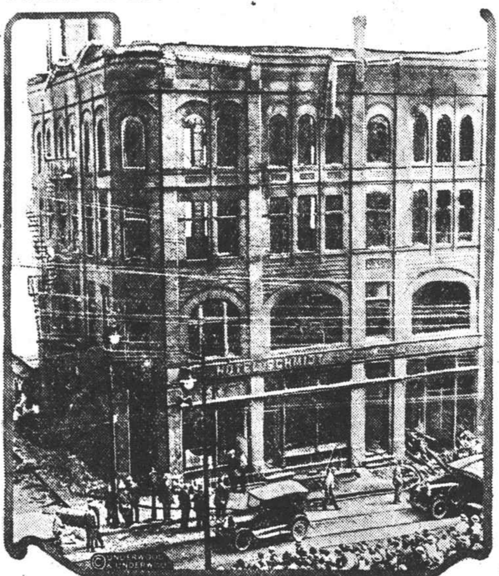
This shows the ruins of Hotel Schmidt, McKeesport, Pa., near Pittsburgh, where four persons are known to have lost their lives and where others may have perished.
