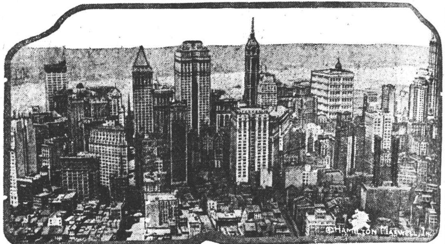
The bulk of the world's wealth is handled here. The famous streets we hear so much about can be seen plainly. To the left is the narrow street called Wall Street; looking west toward Trinity church, the Bankers' Trust building is seen with its pyramid top. A little over toward the right are the Equitable building, the Singer building and the Woolworth.
