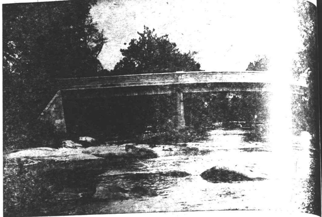
BRIDGE OVER FRENCH BROAD
