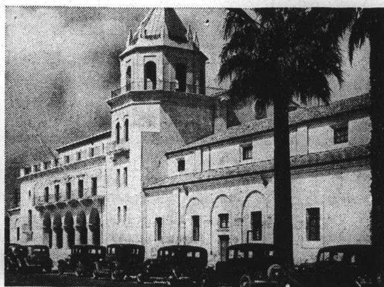
Here, beautifully situated amid palms, is the new municipal auditorium in San Jose, Calif. It was erected with the aid of a PWA grant of $500,000, and is the first unit of the city's proposed civic center. Other imposing buildings are expected to form a part of this new development, which will make San Jose one of the most imposing cities of California.
