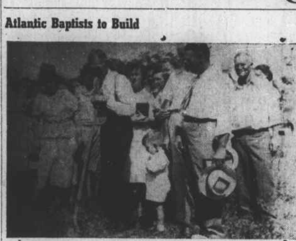
Thomas Nelson, using the spade, breaks ground for the new Baptist church at Atlantic. The ground breaking service was held early last month. Standing to the right of Mr. Nelson is the Rev. L. C. Chandler, pastor, at the extreme right, O. C. Lawrence, contractor. Members of the congregation are in the background.
