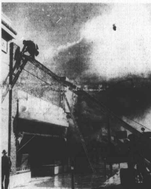
From Beaufort's ladder truck, firemen clambered hour after hour to the rooftops, carrying with them hose through which tons of water flowed.
