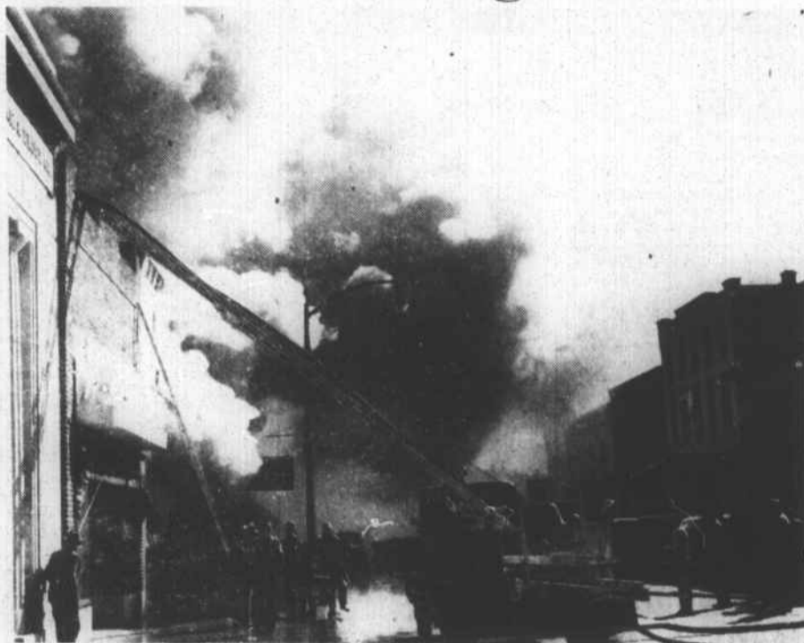
Repeated monstrous puffs from the three burning buildings, Rulane, Downum's 5 and 10, and Downum's department store, blanketed Front street intermittently with yellow smoke that obstructed visibility and made breathing practically impossible.
