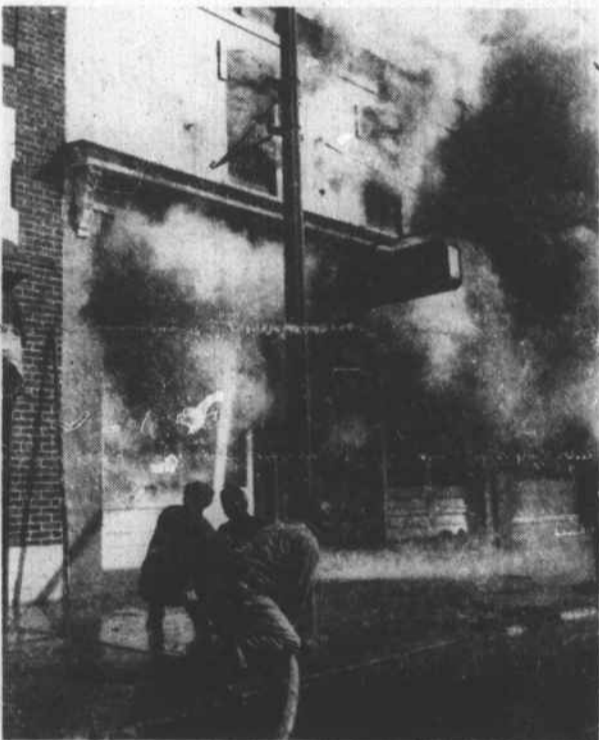
Beaufort firefighters train a hose upward from the sidewalk as heat subsided about noon, allowing them to get closer to the source of the blaze. This shows the front of Eastern Rulane. Today the store is boarded up to prevent the curious from wandering among ruins and being trapped by charred timbers or walls in danger of collapsing.
