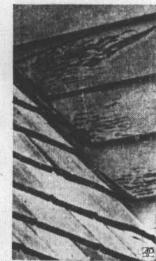
Poor quality paint, left, does this. The U. S. Forest Products Laboratory found no evidence of cold weather condensation or other inner mosture on this job. Poor carpentry, right, causes this. Split clapboard near top has absorbed rain. Other boards, carelessly cut, touch roof. All boards should have been cut slightly shorter and their ends should have been primed. Then adequate flashing would protect paint.
