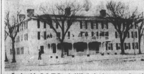
Purchased by C. S. Wallace in 1907, the hotel name was changed from New Bern House to the Hotel Charles. A double porch extending across the front and on one end was removed, being replaced by a smaller porch which extended over the walk. The chimneys were of unusual construction. Each contained six separate flues which connected with fireplaces. This picture was made in 1908.
