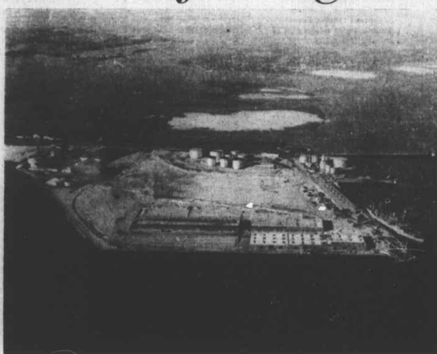
The new Morehead City port, combined with facilities built 17 years ago, features 2,550 lineal feet of wharfage. Two storage warehouses contain 88,000 feet of storage space, two transit sheds 92,000 feet, with paved open storage totaling 60,000 feet. Photo by Jerry Schumacher
