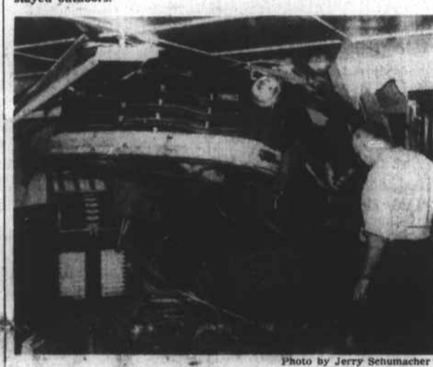
Here he looks over the part of the truck that crashed through his front wall. Fortunately, no one was injured in the wreck, not even the driver.
