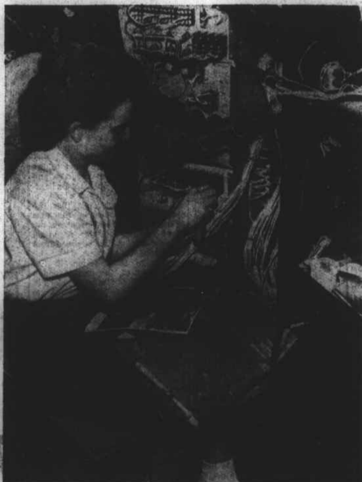
6. Skilled girl worker installs intricate electrical wiring system. She uses blueprint and photograph for reference to installation procedures.
